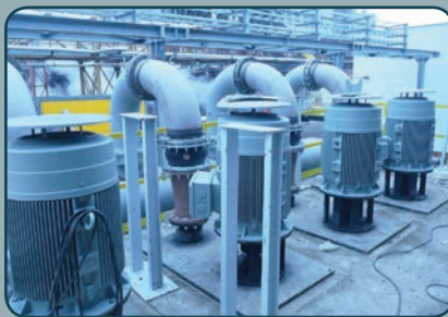
PREOL a.s., COOLING CENTRE, PUMP UNITS CSEV SERIES – VERTICAL VERSION WITH 132 KW MOTORS
