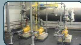
MEROCO a.s., FAME PRODUCTION, PUMPS CSM SERIES WITH MAGNETIC COUPLING
