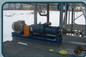
NCHZ a.s., PUMPING OF PROPYLENE-OXIDE, PUMP UNIT CMM SERIES WITH MAGNETIC COUPLING
