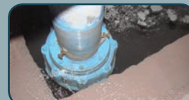
U.S. STEEL KOŠICE s.r.o., ABRASIVE MEDIA, PUMP UNITS CSX-V SERIES CANTILEVER
