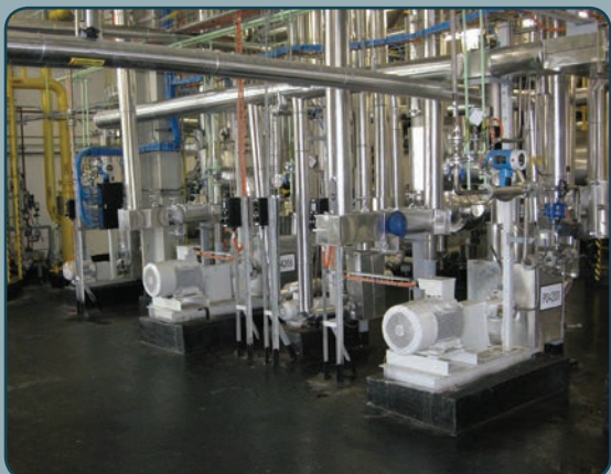
PREOL a.s., FAME PRODUCTIONS, PUMP UNITS CSI WITH HEATED JACKET
