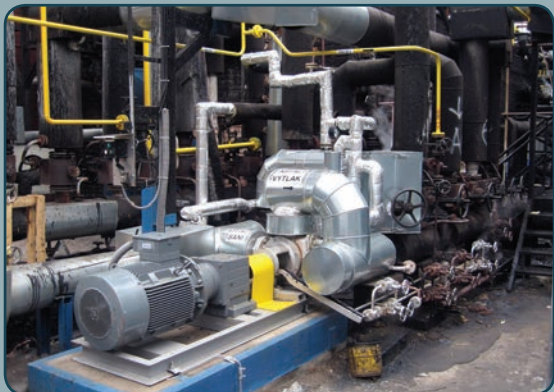
PARAMO a.s., ASPHALT, PUMPS MV SERIES WITH HEATED JACKET
