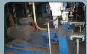
VÍTKOVICE a.s., PRESSURE BOOSTING IN PROCESS TO 80 BAR, PUMP UNITS CSA SERIES, STORAGE OH2
