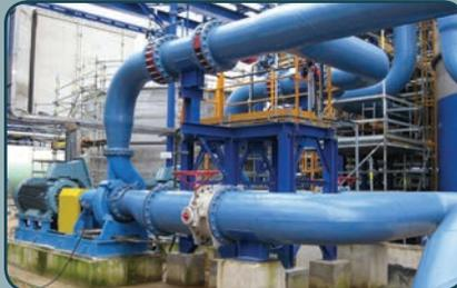
GPN S.A. (FRANCE), PRODUCTION OF NITRIC ACID, PUMP UNIT CSO SERIES WITH 500 KW, 5500 V MOTOR
